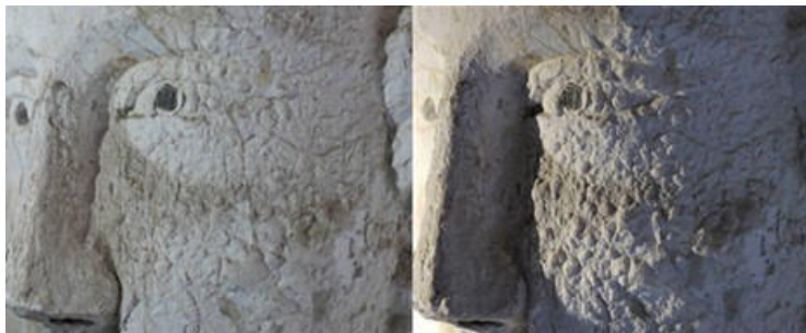
Figure 1 - Particular of the deterioration of the capital in Vis diffuse (left) and grazing (right) lighting
